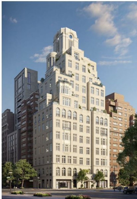
The new condominium on Madison Avenue is designed to look like a prewar building. Source: Compass
